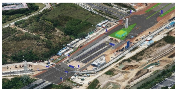
图4 查看地下道路入口情况 Fig 4 View the entrance of the underground road
